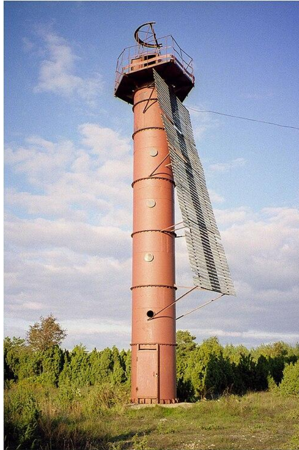
Figure 17 A daymark tilt backwards for better illumination (Sviby rear leading mark by Tuderna, licence CC BY 2.5.)
